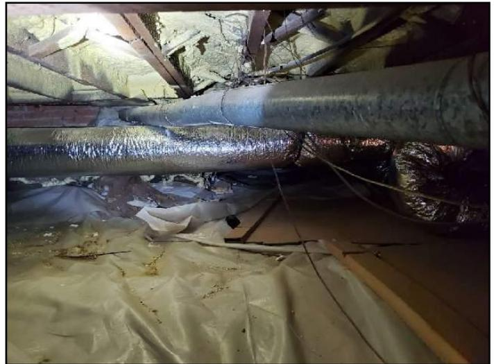
**47. Condition:** • The water heater vent pipe is corroded and holes were noted in the crawl space. This is a significant safety concern that should be addressed promptly.
