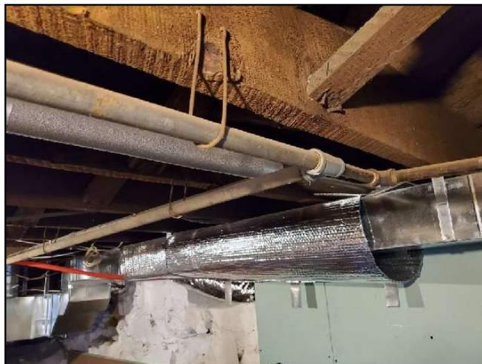
**43. Condition:** • No gas isolation valve was found for an appliance. If there is no isolation valve, one should be installed by a licensed plumber. If there is a valve that is hidden it should be made accessible.
