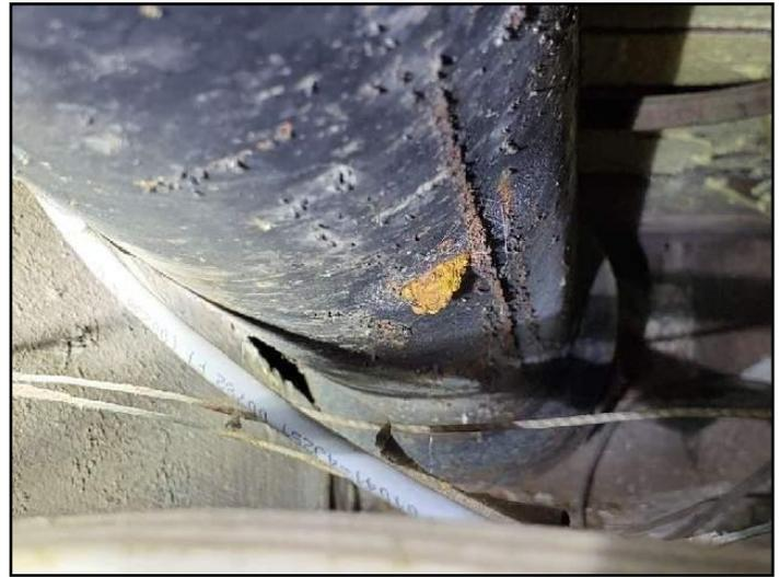
**50. Condition:** • The cast iron waste pipe in the center of the basement is split and should be replaced.
