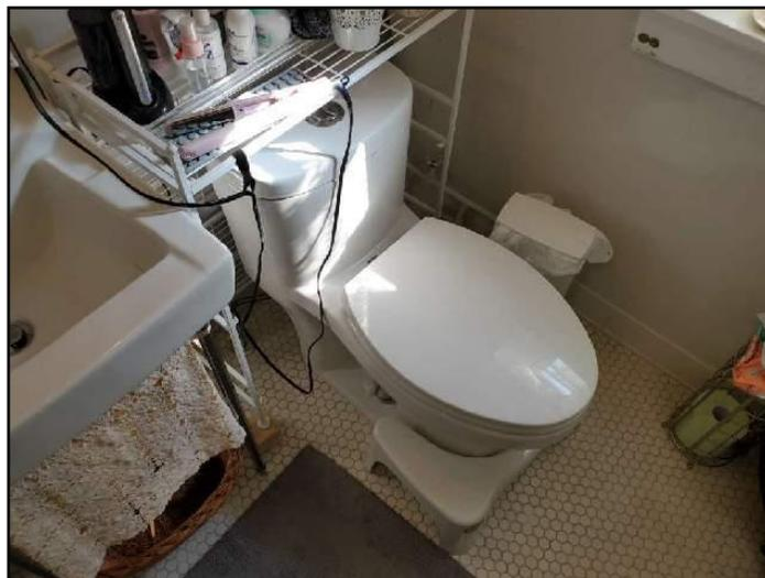
**57. Condition:** • The toilet runs on after flushing. I recommend replacement or adjustment of the flush valve assembly to eliminate the leakage.
