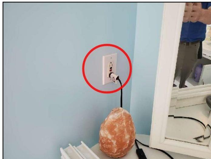
**30. Condition:** • Improperly wired outlet(s) (e.g. reversed polarity or ungrounded) should be investigated by a qualified electrician and repaired as necessary.
