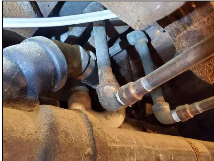
**41. Condition:** • I recommend capping any open plumbing supply pipes to reduce the risk of leakage if the valve does not remain closed completely.
