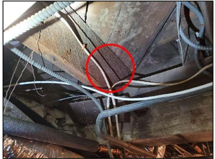
**22. Condition:** • A cut joist was noted at the center of the basement (front of the center beam). The repair to the joist is insufficient. The joist should be properly repaired/supported.
